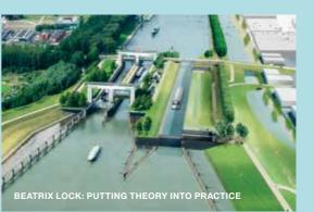
on the Beatrix lock project (the Netherlands), virtual reality was used to create an environment which could be visited by maintenance technicians, allowing them to provide their aput early on in the design process in order to optimise the naintainability of the lock doors. The VR model was connected to the command and control system, giving the traffic nanagers of our client a 100% realistic experience of the functionality and UX (user experience) of the future lock.
